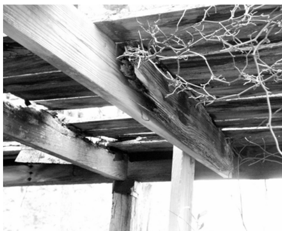
Figure 8 View under north end of rear deck, showing remains of original floor framing. (NPS-SERO-CRS, 2001)
