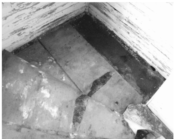
Figure 15 View of floor in northwest corner of main room, showing early felt-based, imitation linoleum under two later floor coverings. (NPS-SERO-CRS, 2001)
