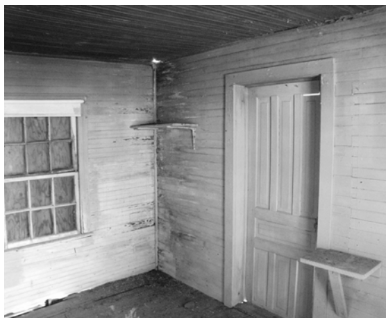
Figure 17 View south in Room 101. Door to right was originally a window opening, converted into a door to the addition in the 1950s. (NPS-SERO-CRS, 2001).
