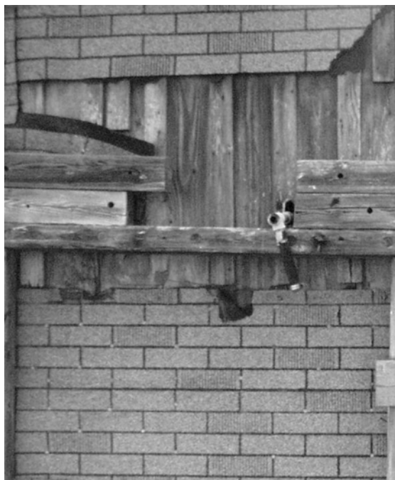
Figure 11 View of “brick” asphalt-composition siding over original board-and-batten siding at northeast end of house. (NPS-SERO-CRS, 2001)
