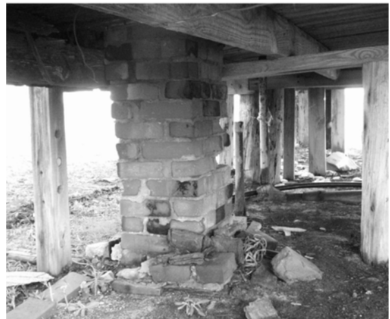
Figure 16 Top, view of chimney stack; below, view of chimney foundation. (NPS-SERO-CRS, 2001)
