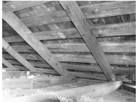
Figure 9 View of southeast shed of roof; note wood shingles still in place. (NPS-SERO-CRS, 2001)
