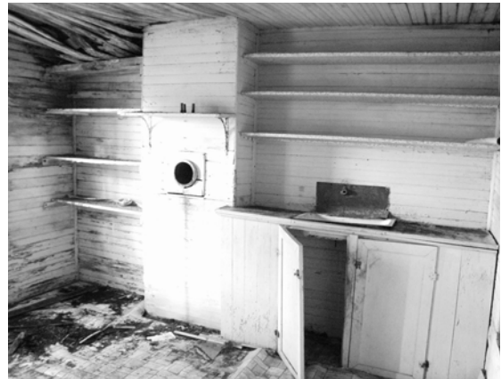
Figure 12 View north in main room (101). Sink is to right of chimney. (NPS-SERO-CRS, 2001)
