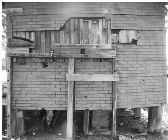
Figure 3 View of remains of wooden frame for cistern at northeast end of house. Parts of a brick foundation remain in the ground below. (NPS-SERO-CRS)
