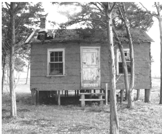
Figure 2 Left, view southeast of front of Styron House. (NPS-SERO-CRS, 2001)
