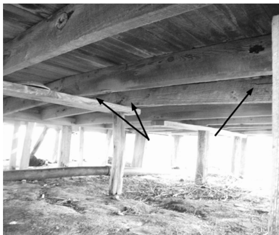
Figure 7 View of floor framing; arrow at right indicates where joist has split; arrows at center show location of two joists that have broken where they cross the added support beam. (NPS-SERO-CRS, 2001)
