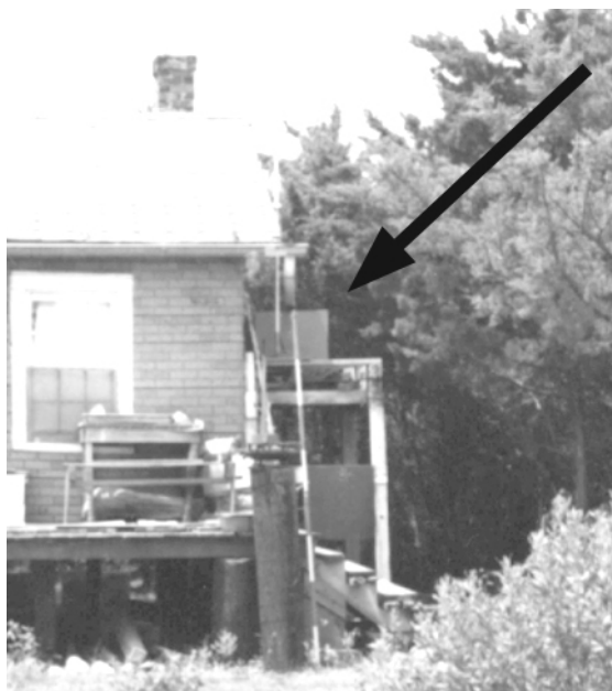
Figure 18 Detail from 1984 photograph, with arrow indicating now-missing cistern. (NPS-CALO, 1984)
